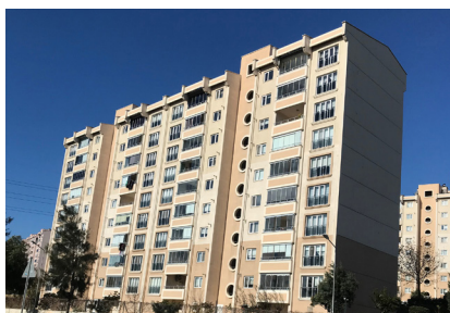
Building B's natural gas heating bill is on average 3,211 euro per year, 30% more!
