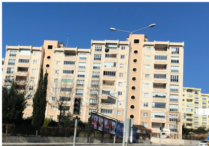
Building A's natural gas heating bill is on average 2,470 euro per year.
